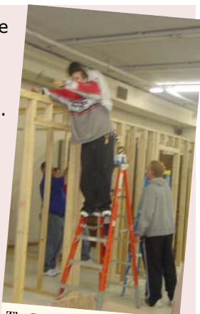
The Person High School Carpentry Class at work building office space
