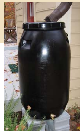
The barrel is positioned under a gutter and stationed on an above ground object such as cinderblocks. Sells for $80.00.
